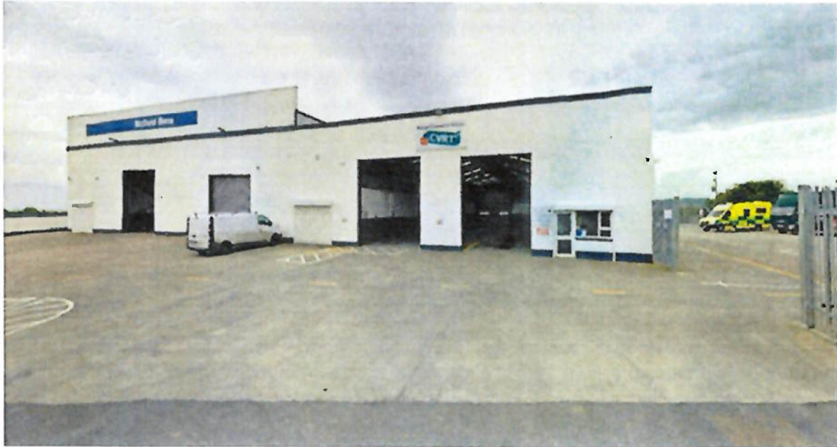
Front of premises – view from existing N13
