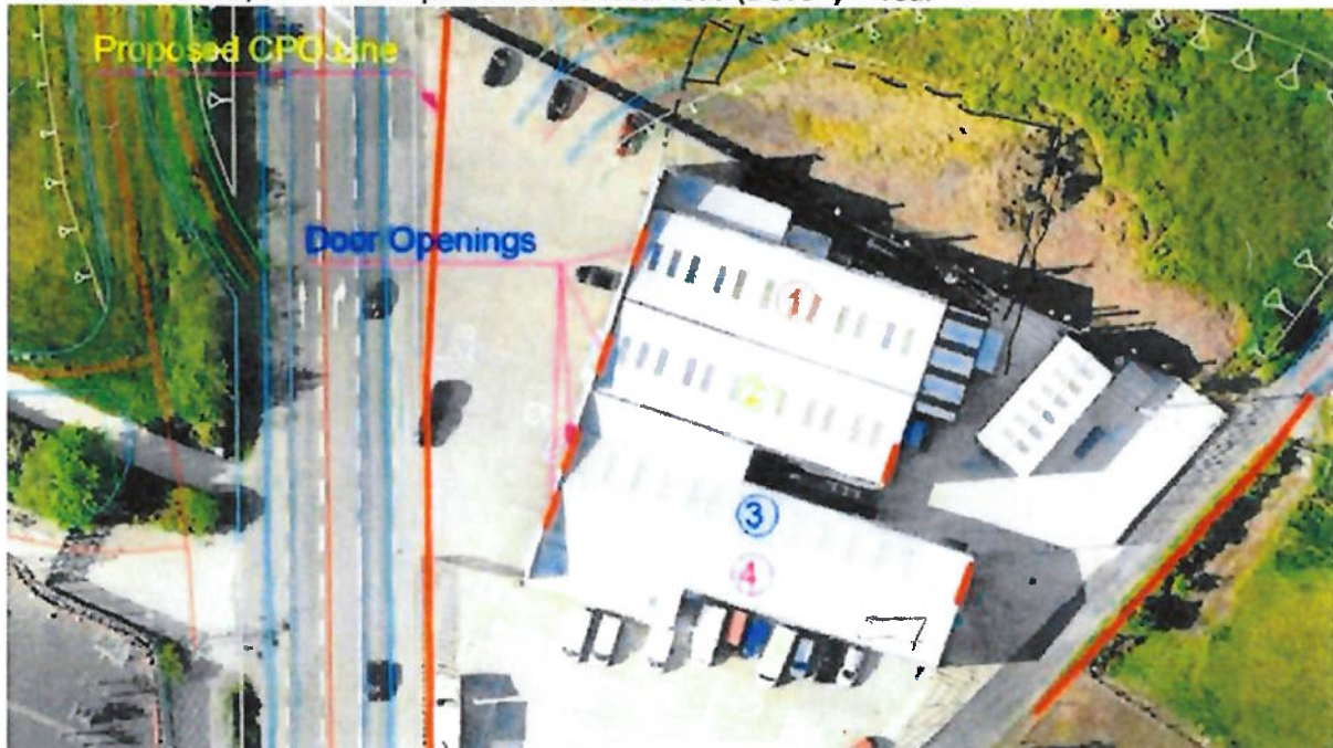
Aerial view of N13, commercial premises and local road (L-5794) in rear
